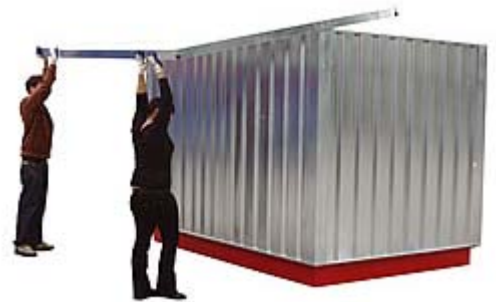
6. Slide on the roof
