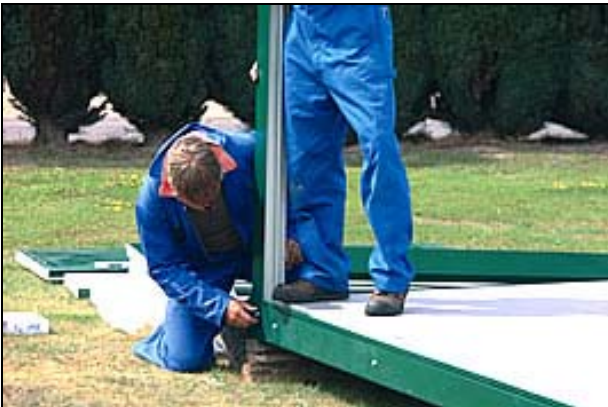
Fix the four corner posts
