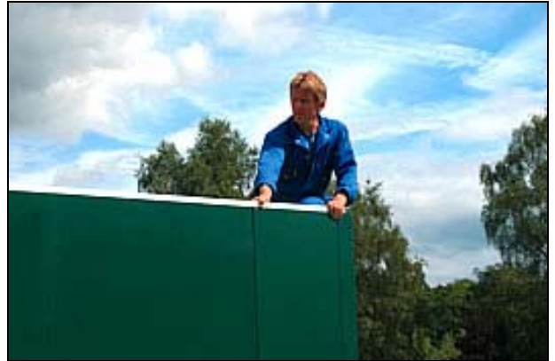
Fit the ceiling retention bars
