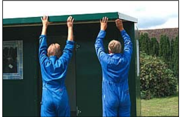
Fit the outer roof skin
