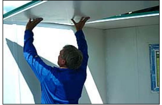
Slide in the ceiling panels
