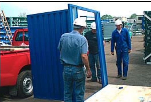
Fit panels to the Expandastore base
