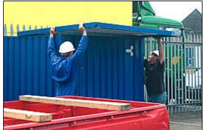
Lift on & fix the roof
