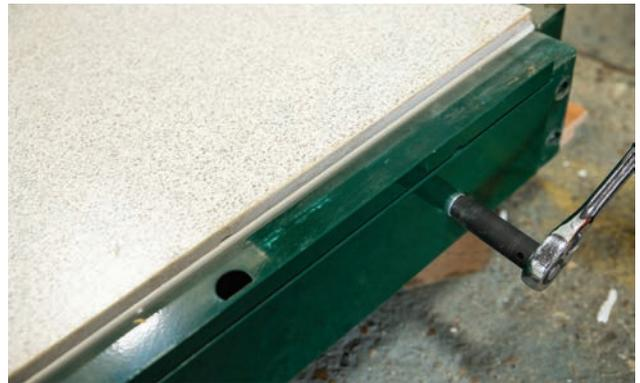
5. Reassemble floor at your planned erection location.
