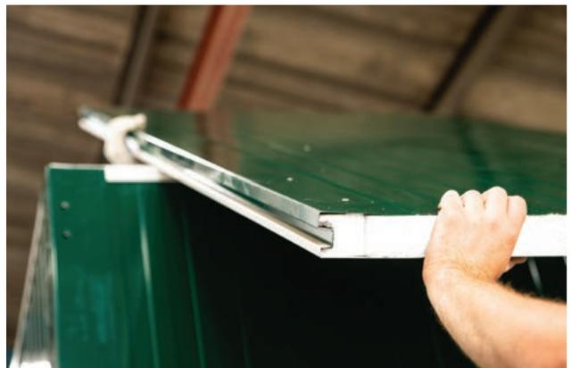
13. The ceiling panels join in a similar way to the wall sections. Fit the H section joints but please note that the grey box joint needs to be laid in place before fitting the next panel (rather than sliding in afterwards). When it comes to fitting the final roof panel you may need to push the panels up in the middle of the cabin by using the stepladder to align the panels correctly between the end panels.
