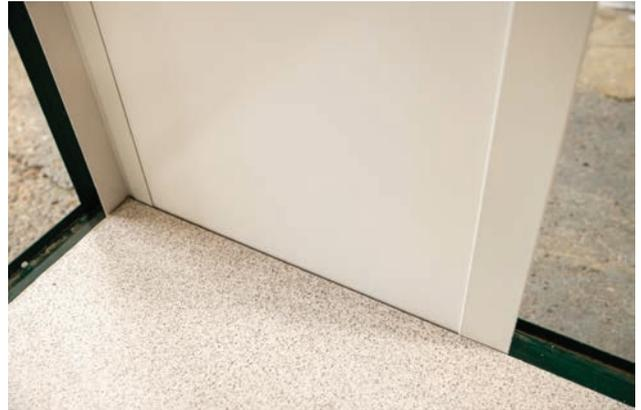
5. Now slide in the next panel, interlocking the tongue and groove joint.
