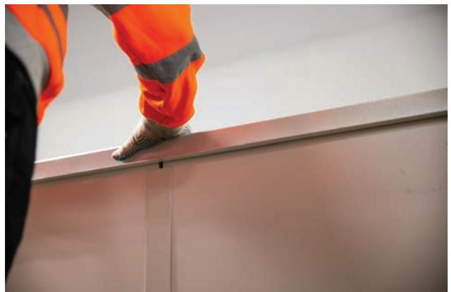
12. Use the stepladder to do this. These sit inside the ceiling. The lip on the top rail needs to be on the inside of the cabin.
