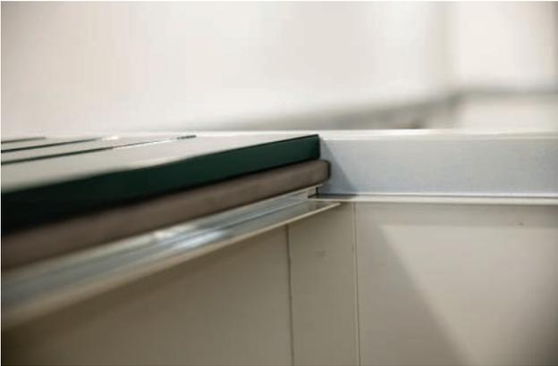
14. Slide on the roof section by lifting onto the shortest office side and then sliding up. You will need at least four people and two stepladders to carry this out safely. If space is tight, it can also be slid up from the side but you may need some extra help.
