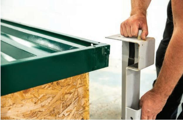
2. Remove the roof panel and set down
