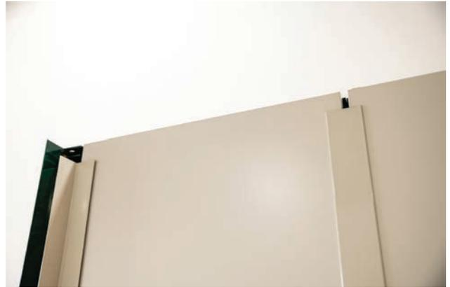
6. Using your stepladder, from the top of the panel, slide one of the grey plastic box section joints down from the top between the wallboards.
