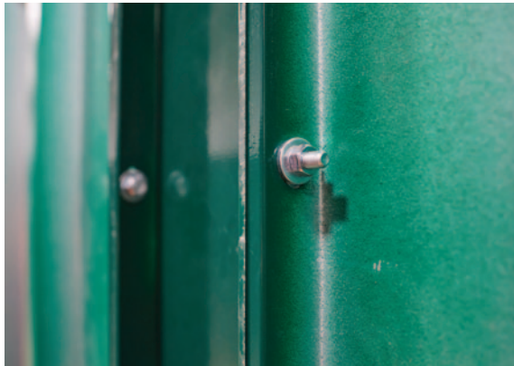
2.19 Secure side panels with M8 bolts.
