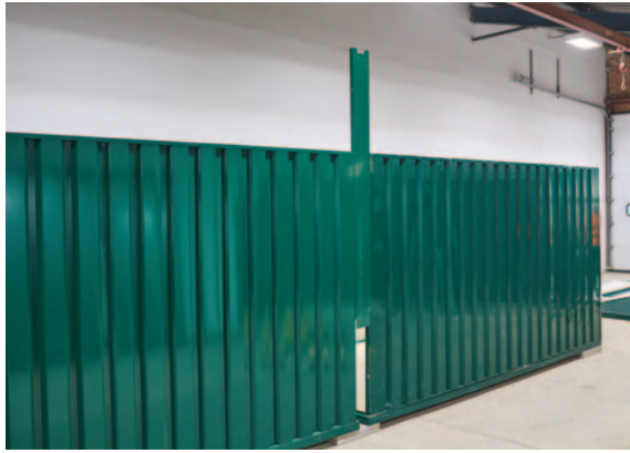
2.18 Fit Side joining strip from above.
